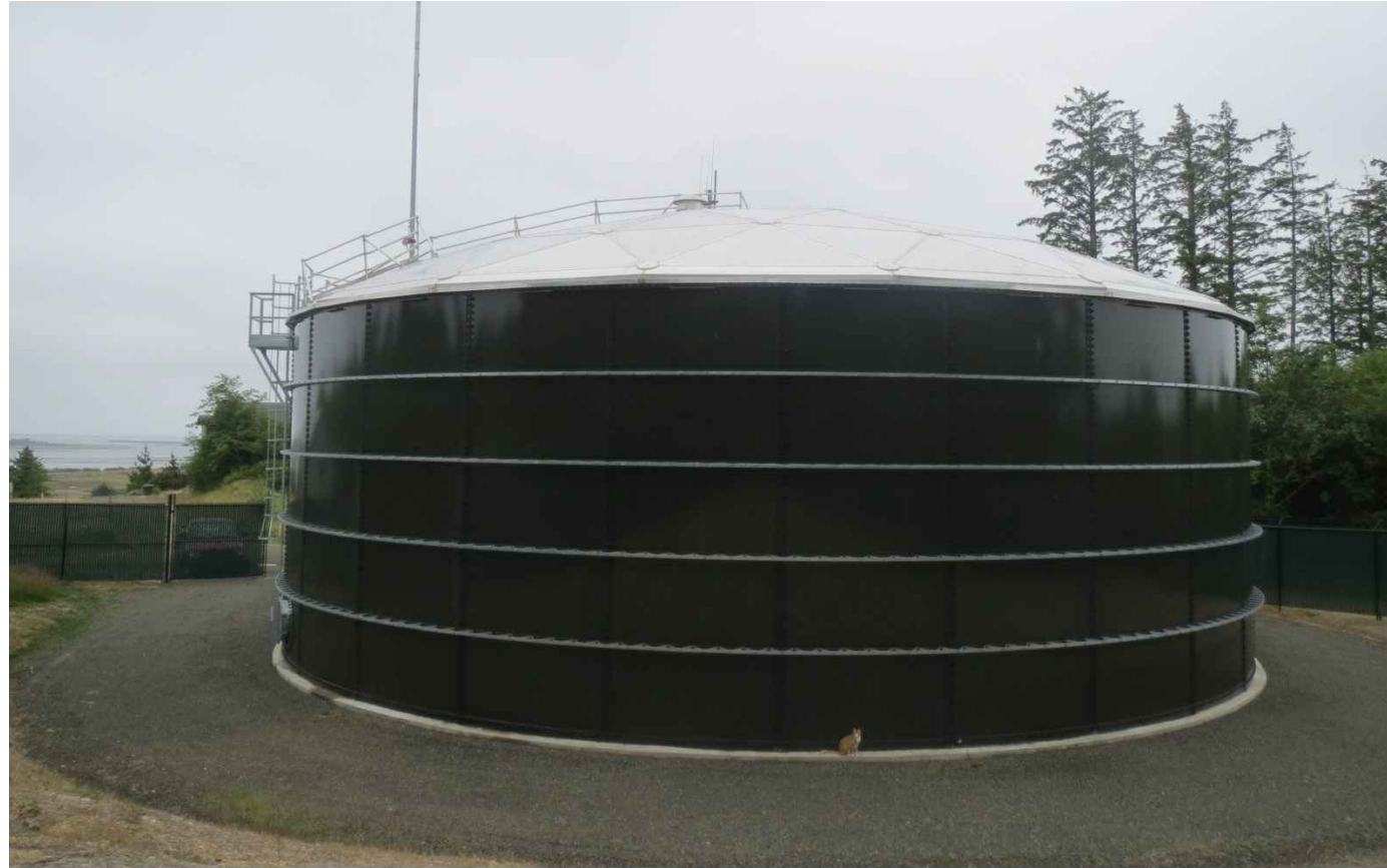
BOLTED STEEL RESERVOIR PHOTO SOURCE: GRAY & OSBORNE
