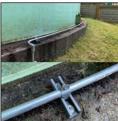
Figure 2: Example of Conduit and Supports along Concrete Footing
