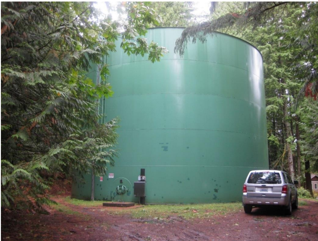
Figure 5: Exterior Division 22 Reservoir
