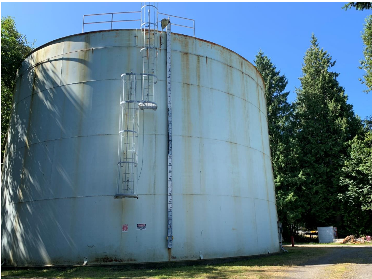
Figure 1: Exterior Geneva Reservoir
