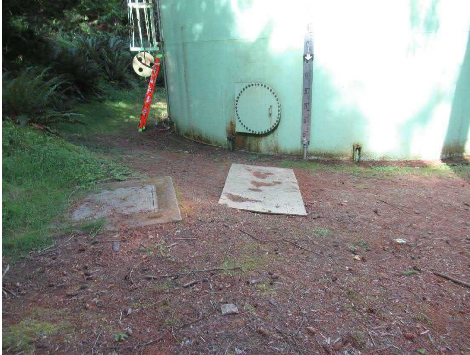
Photo 1: East side of tank.
