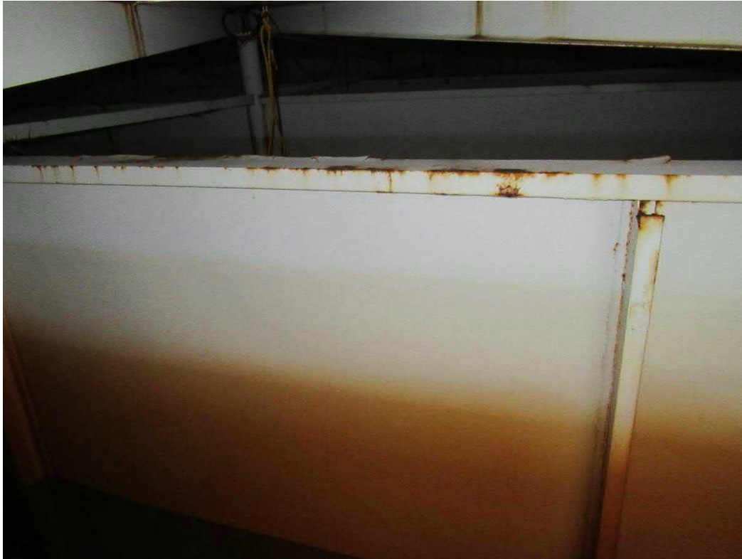
Photo 31: Interior baffle walls.
