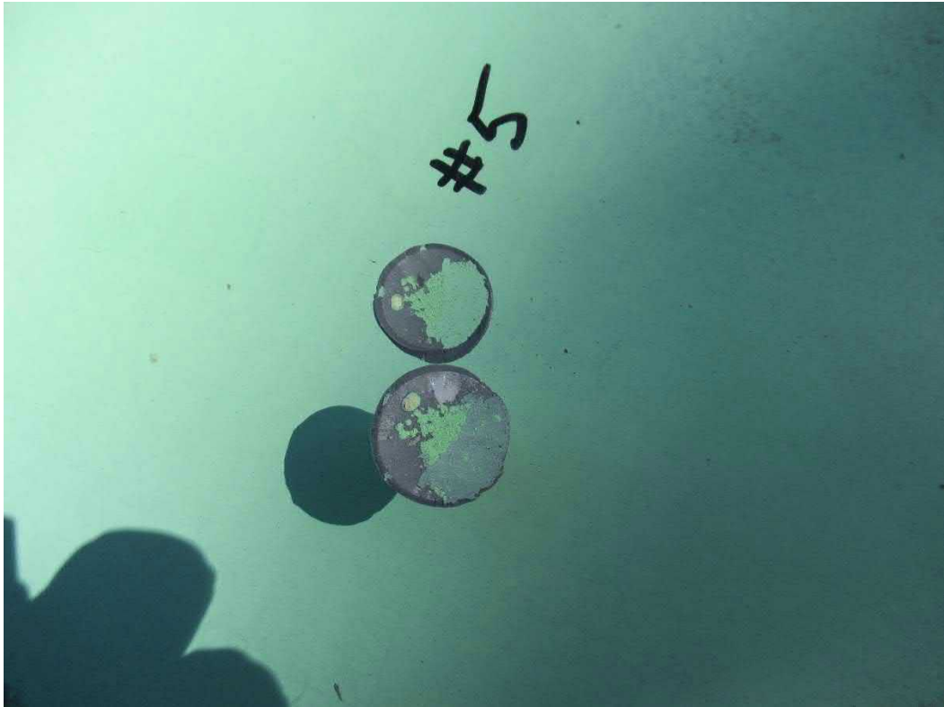
Photo 14: Dolly #5 on the roof.
