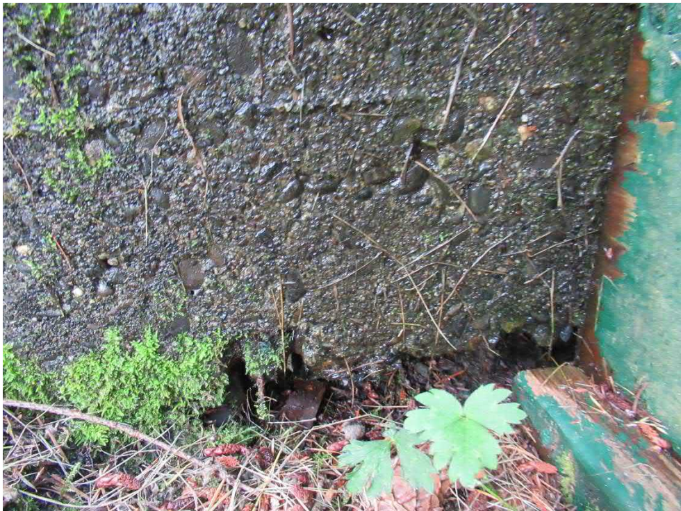
Photo 8: Exposed ring wall on east side by sample lines.
