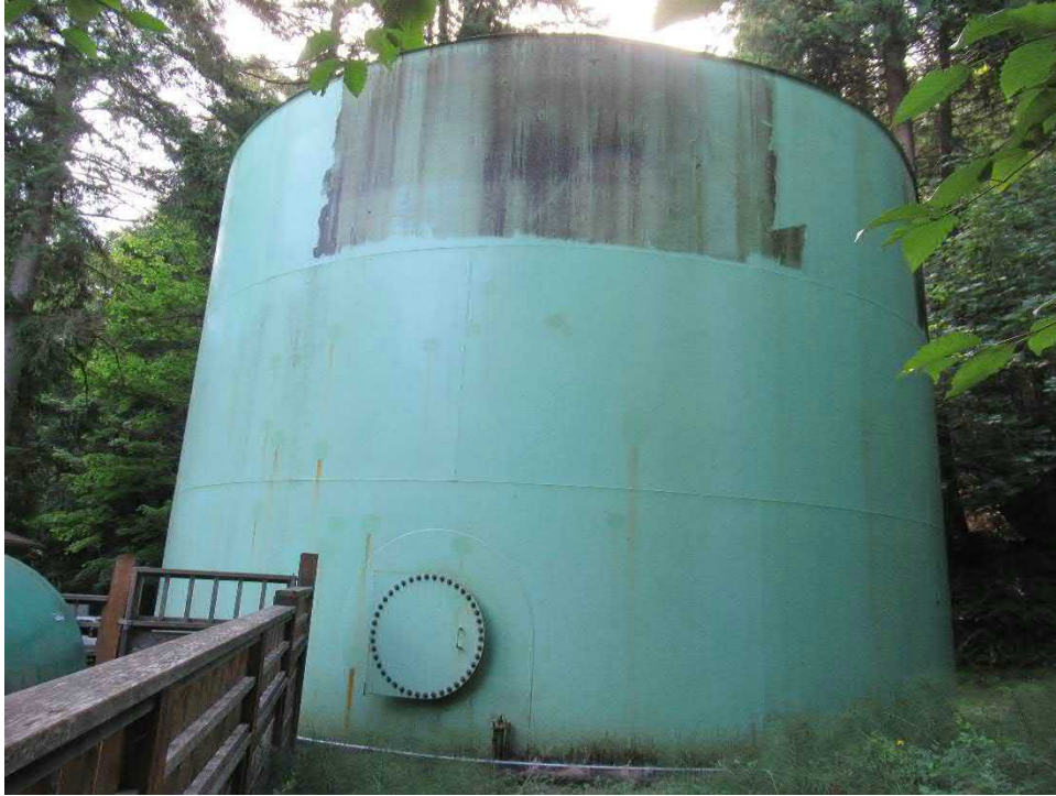
Photo 3: North side of the tank.
