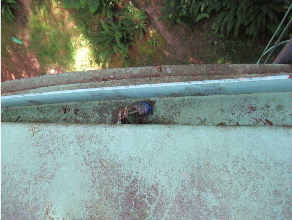
Photo 23: Access hatch lock.
