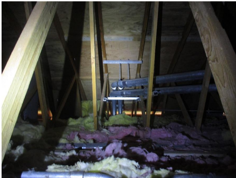
FIGURE B-8 Conduit Runs
