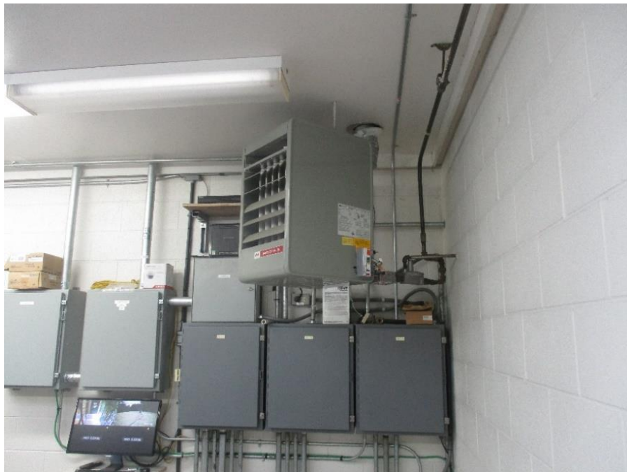
FIGURE B-2 Gas Heating Unit
