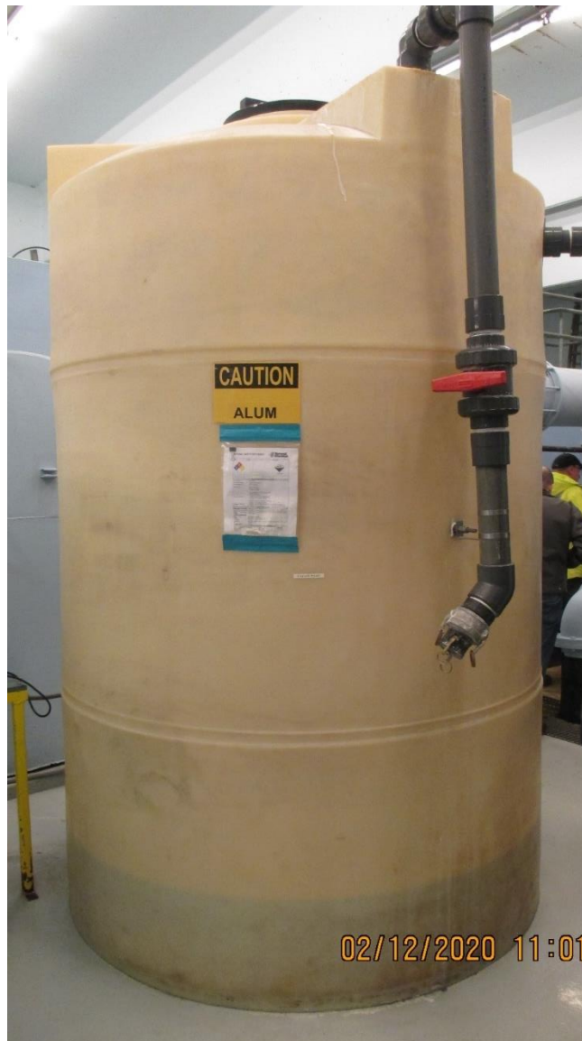
FIGURE A-1 Existing Alum Storage Tank
