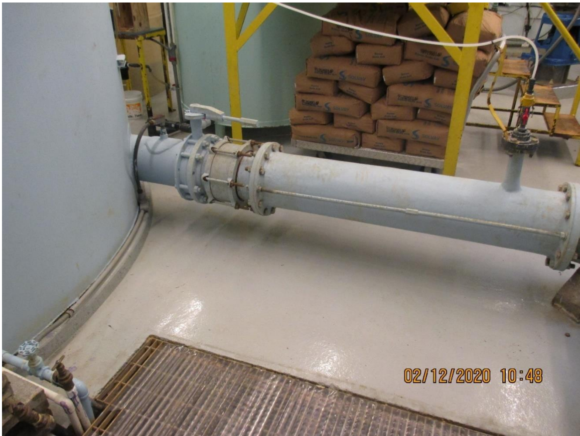
FIGURE A-3 Existing Alum Injection Location
