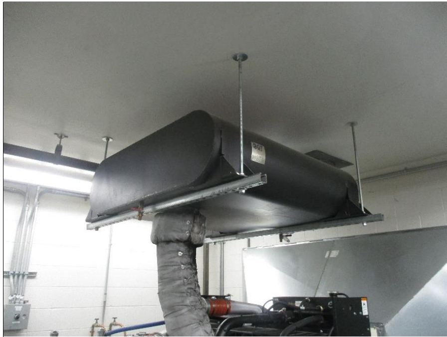
FIGURE B-1 Generator Exhaust
