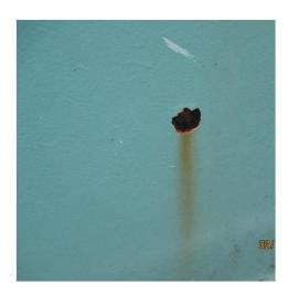
Corrosion – Tank has several corrosion spots, some of which have been repaired.
