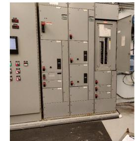
MCC 2 – Located in WTP Main Building. Controls Clearwell Transfer Pumps.
