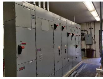
MCC 1 – Located in Finished Water Pump Building. Controls Finished Water Pumps.
