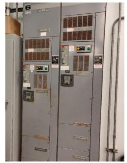
MCC 3 – Located in WTP Main Building. Controls Raw Water Pumps.
