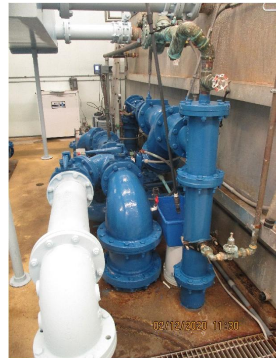
Injection – Lack of features requires daily manual calibration.
