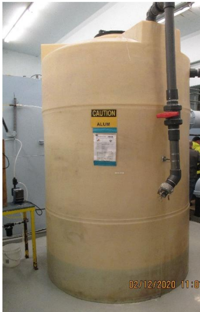
Alum Storage Tank – HPDE. Installed in 1992 and beyond its recommended useful life (15-17 years).
