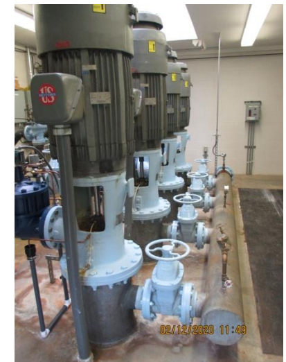
Distribution Pumps – Pumps are original (1990) and near the end of their recommended useful life.
