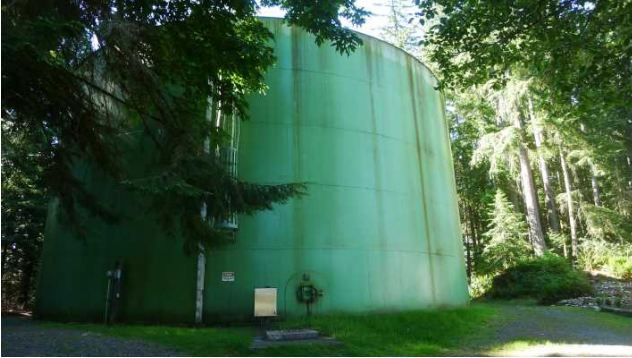
North side of water storage resevoir
