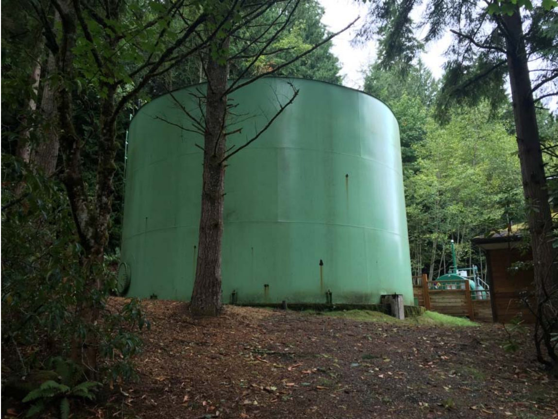
Figure 35 SVWTP Reservoir, September 1, 2015
