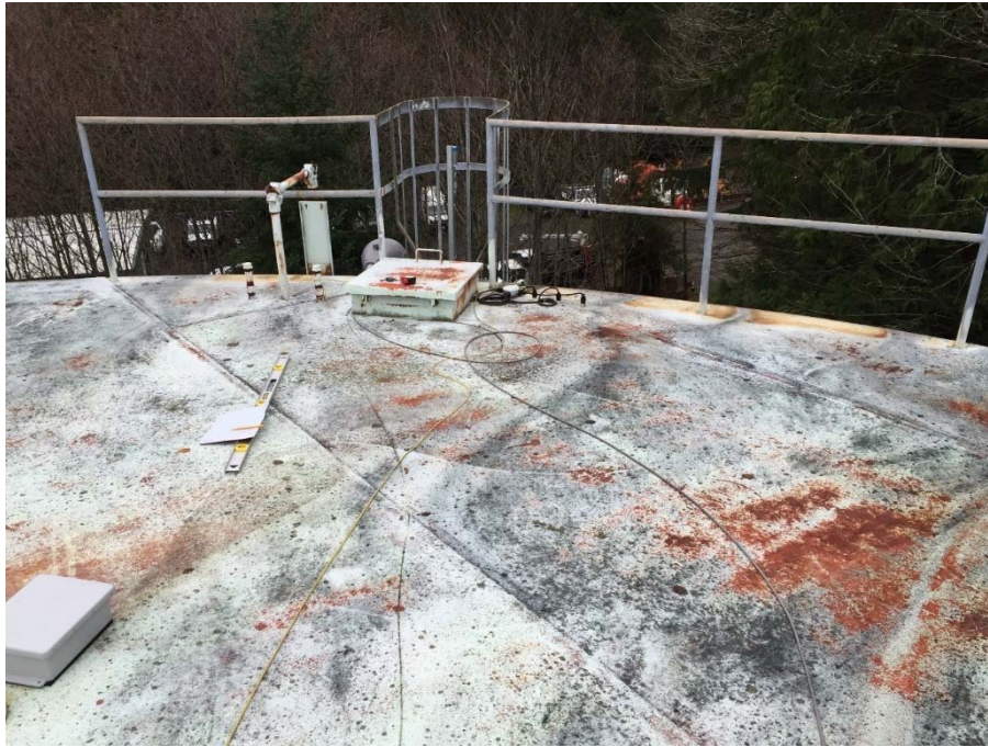
Figure 6 Roof at Entry Hatch
