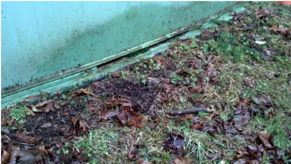
Figure 19 Division 7 Reservoir at Foundation Note missing grout.
