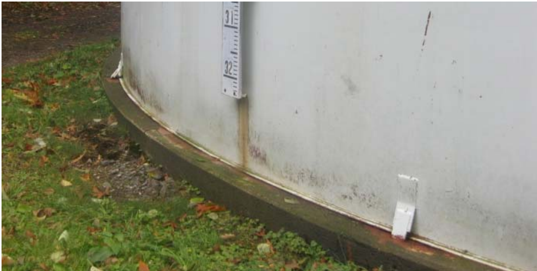
Figure 5 Geneva Reservoir at Shell to Foundation Interface
