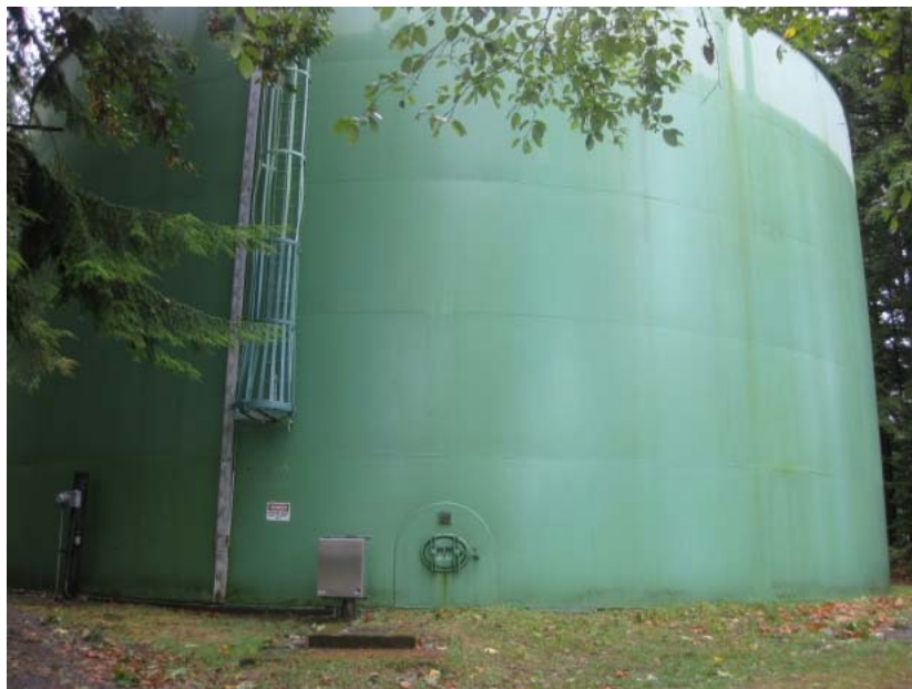
Figure 18 Division 7 Reservoir, September 1, 2015
