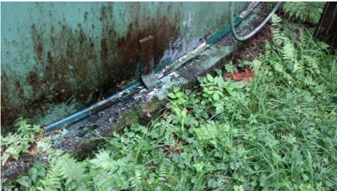
Figure 25 Division 30 Reservoir at Foundation Note typical strap anchor and no grout under the shell.
