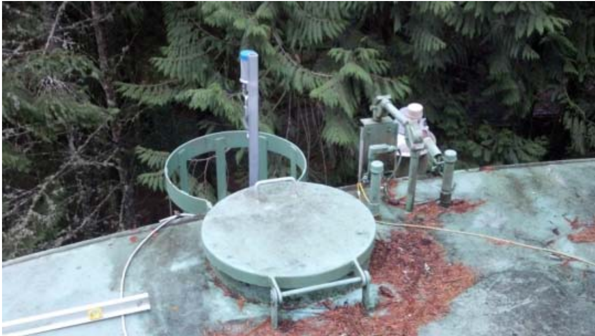
Figure 15 Division 22 Reservoir at Roof Hatch
