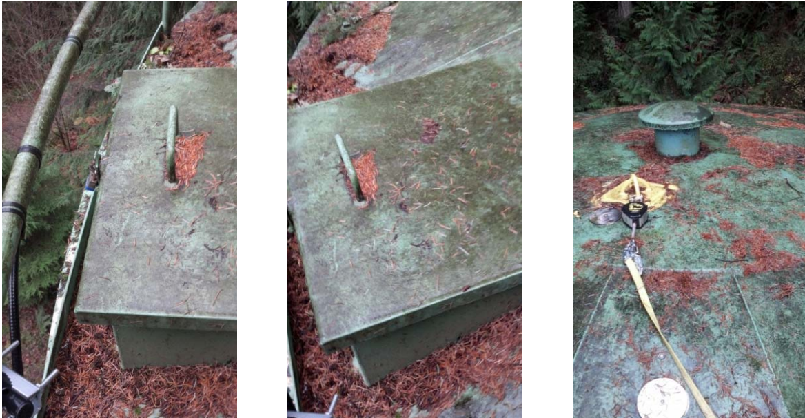
Figures 26, 27, and 28 Division 30 Reservoir at Roof Hatch and Vent
