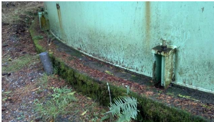
Figure 36 SVWTP Reservoir at Shell to Foundation Interface
