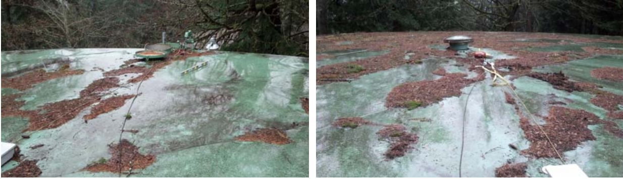
Figures 20 and 21 Division 7 Reservoir at Roof Hatch and Vent
