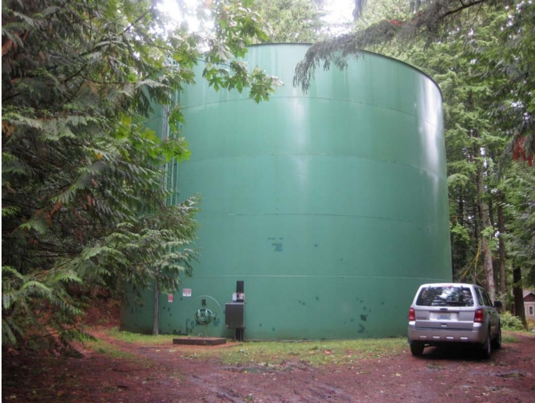
Figure 11 Division 22 Reservoir, September 1, 2015
