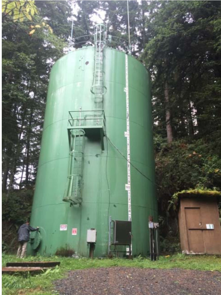
Figure 24 Division 30 Reservoir, September 1, 2015
