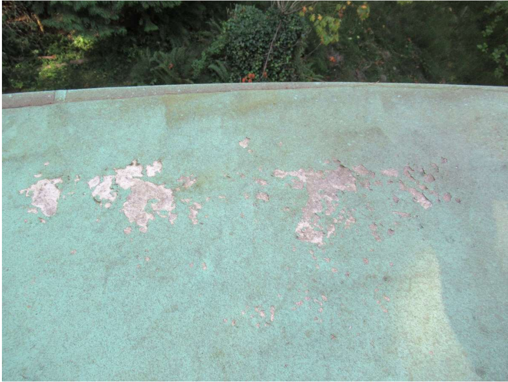
Photo 27: Coating delamination on the roof.
