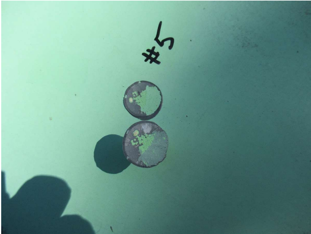
Photo 14: Dolly #5 on the roof.
