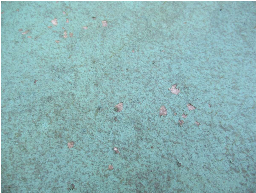
Photo 28: Coating delamination on the roof.
