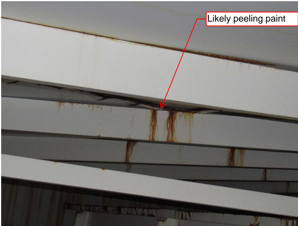
Photo 35: Interior condition. Note delamination in roof.
