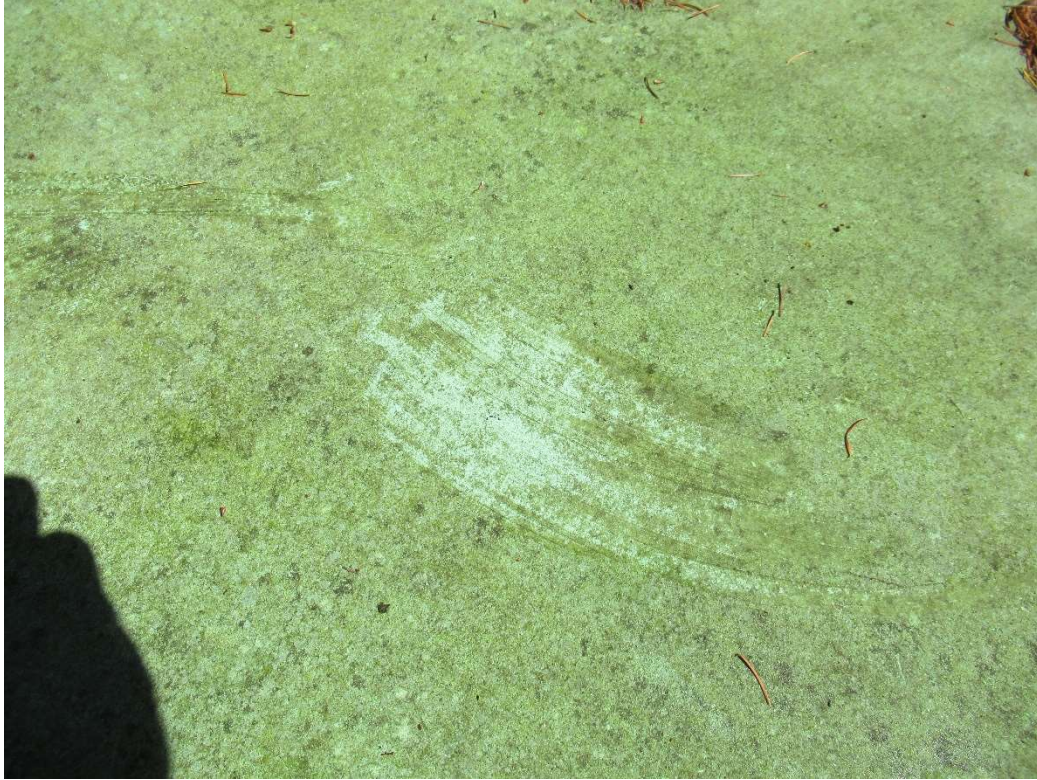
Photo 25: Closeup of the algae on the roof.
