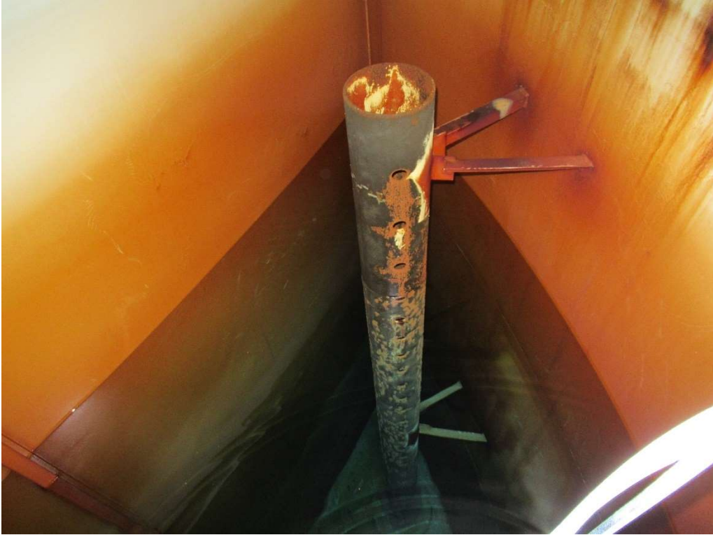
Photo 30: Inlet pipe diffuser.
