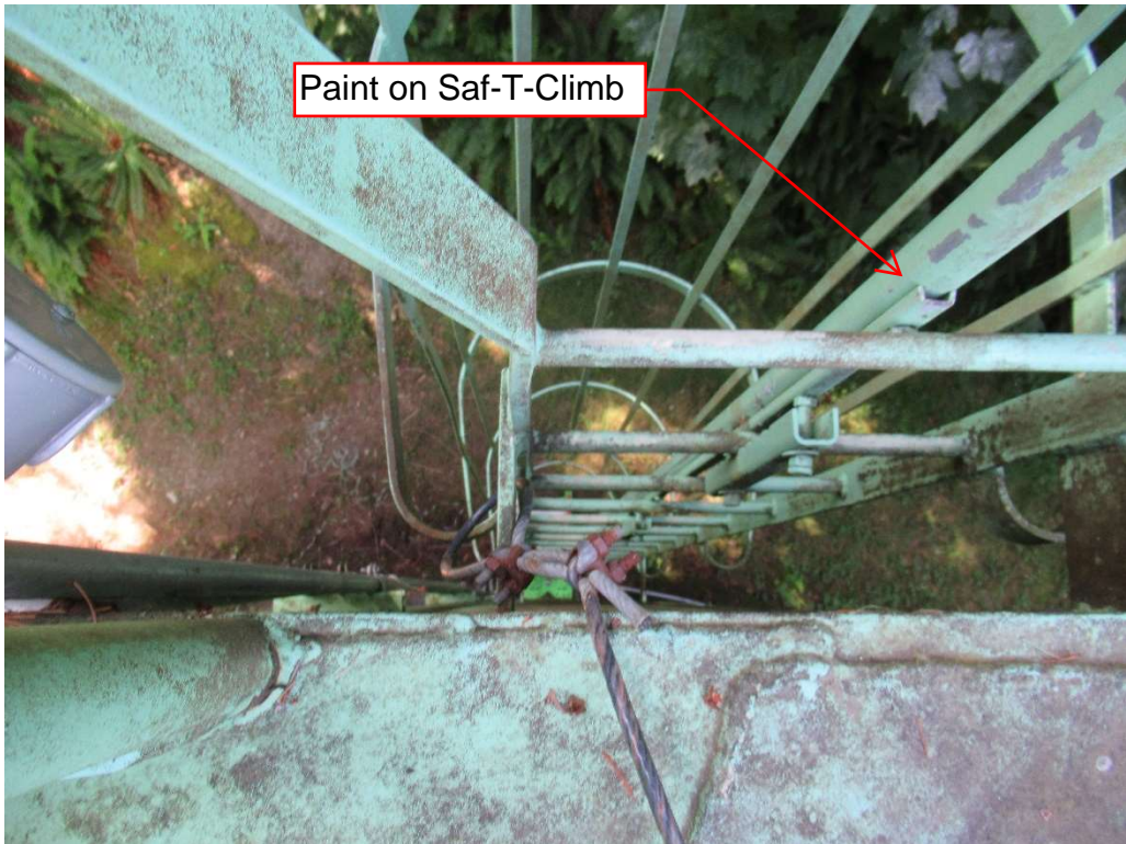
Photo 22: Safety line tied to ladder standoff. Note the Saf-T-Climb is painted.
