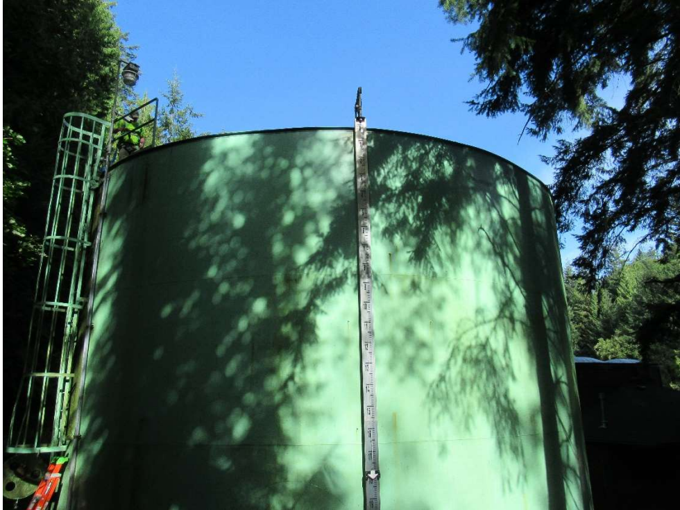
Photo 7: Southeast side of the tank with level gauge.
