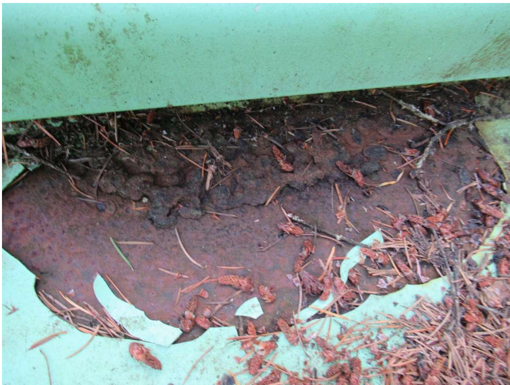
Photo 24: Corrosion adjacent to the access hatch.
