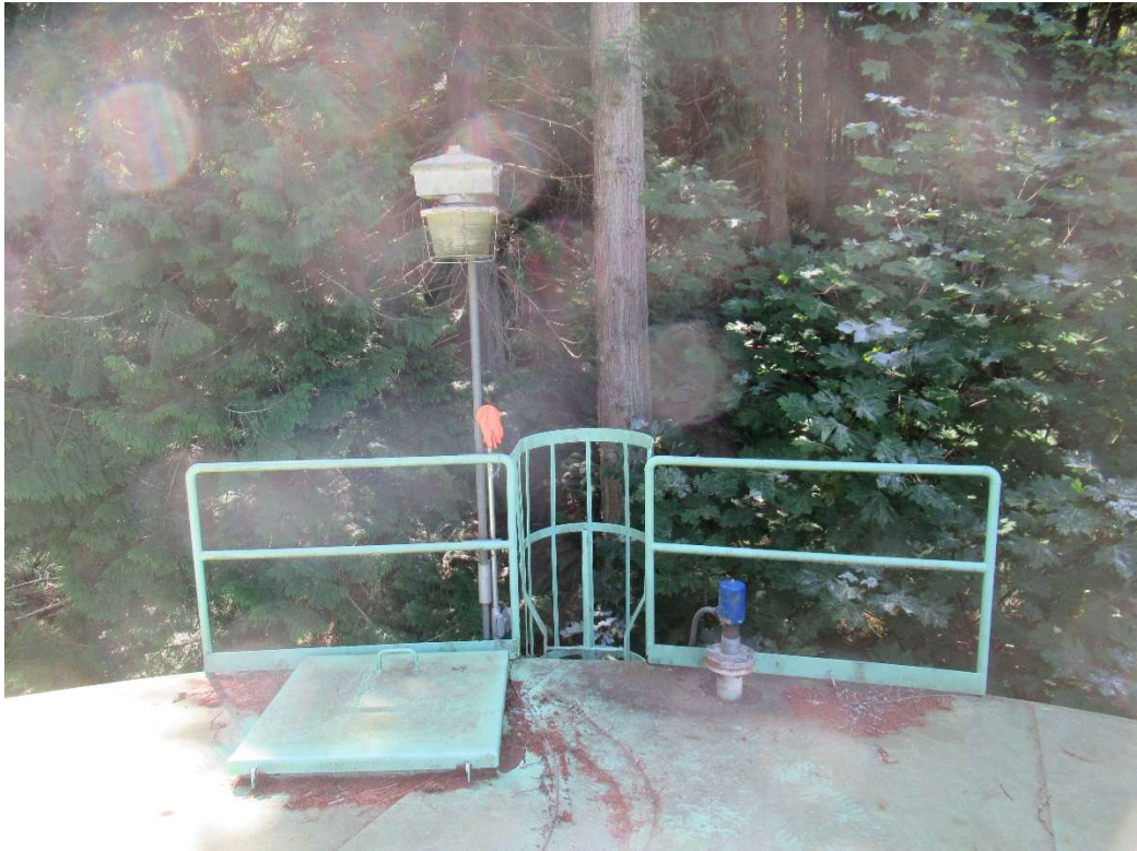
Photo 16: Ladder, railings, camera, and access hatch.
