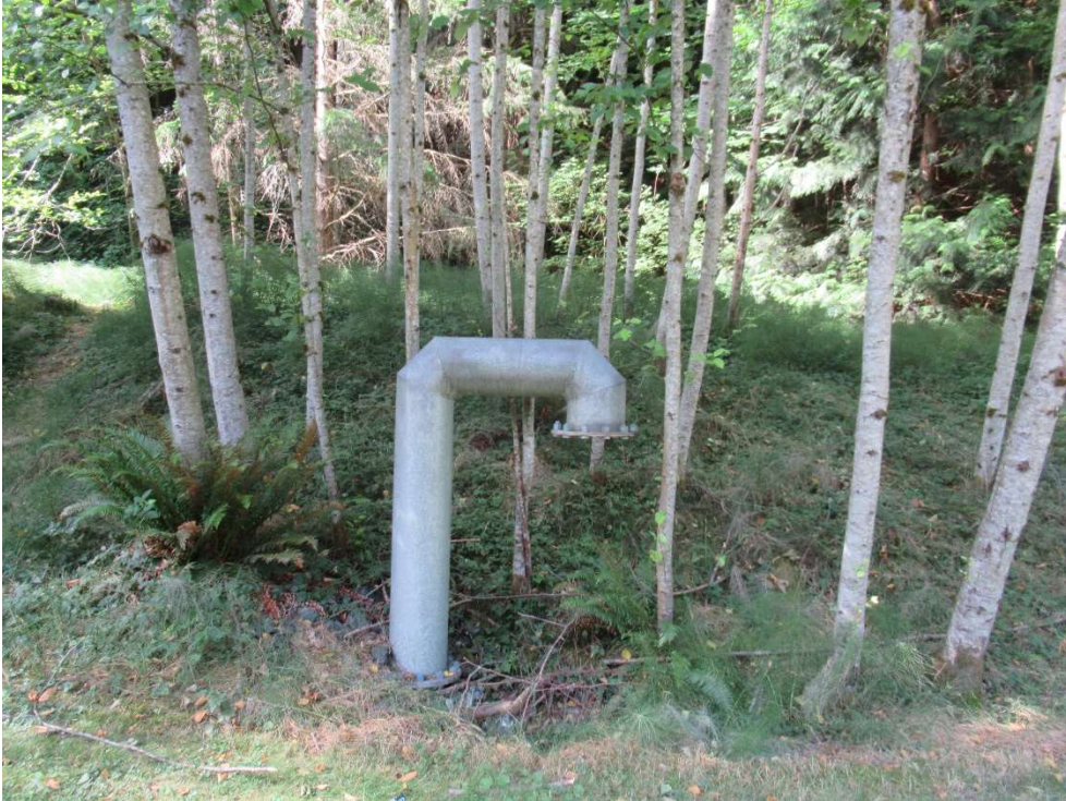
Photo 5: Overflow with air gap.
