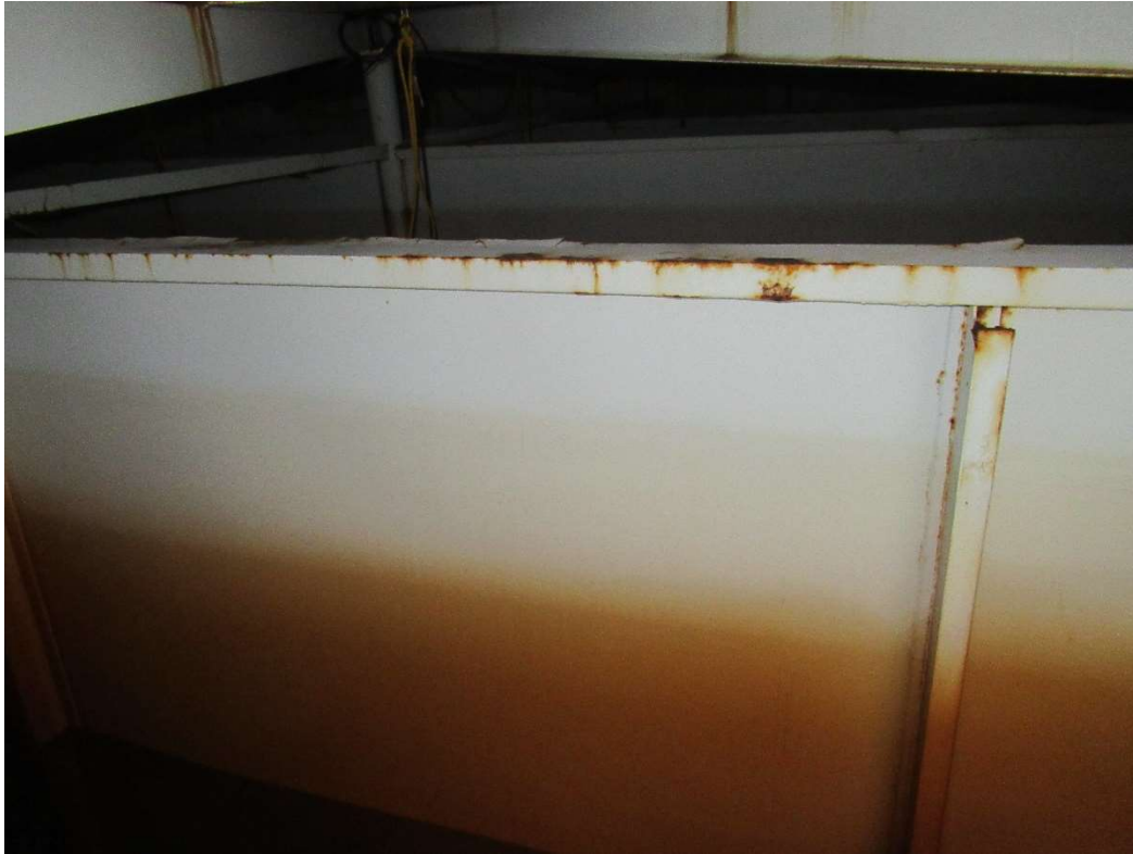
Photo 31: Interior baffle walls.
