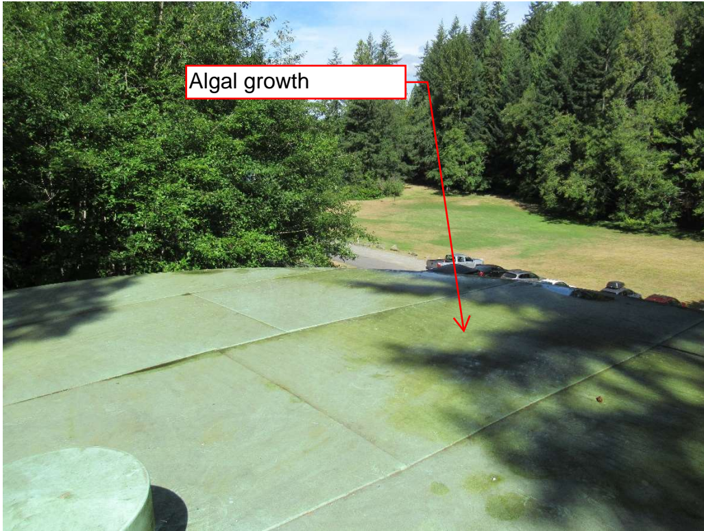
Photo 21: Looking north. Note the algae in the right side of the photo.
