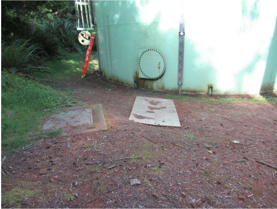
Photo 1: East side of tank.
