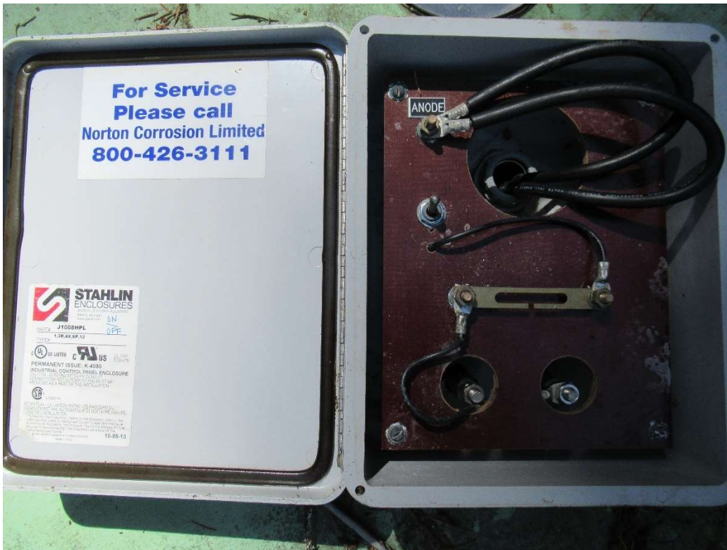
Photo 20: Cathodic protection box.
