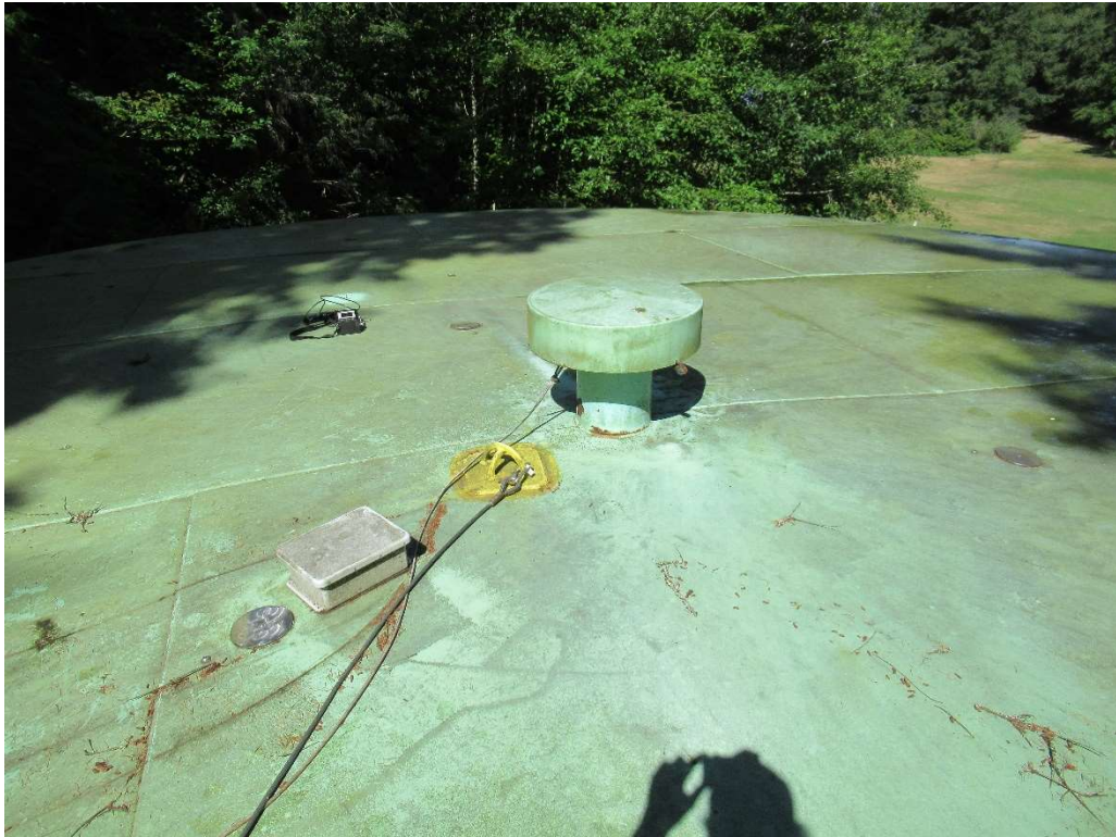
Photo 18: Anchorage, roof vent, and cathodic protection box.
