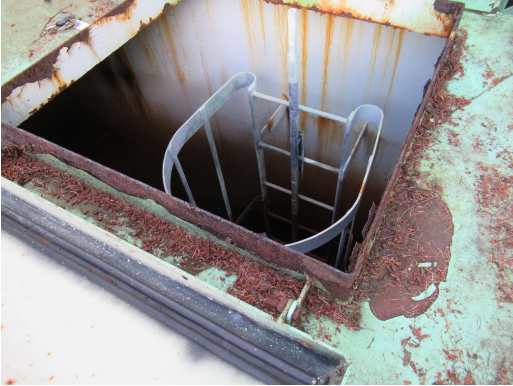
Photo 29: Inside of the access hatch.
