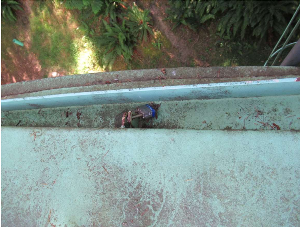
Photo 23: Access hatch lock.
