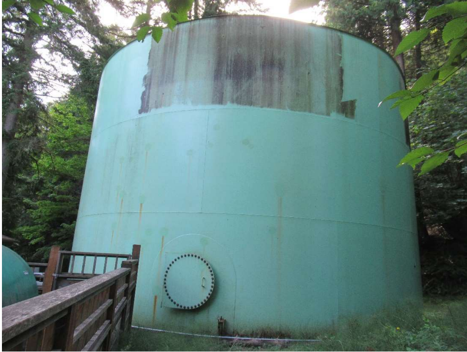
Photo 3: North side of the tank.
