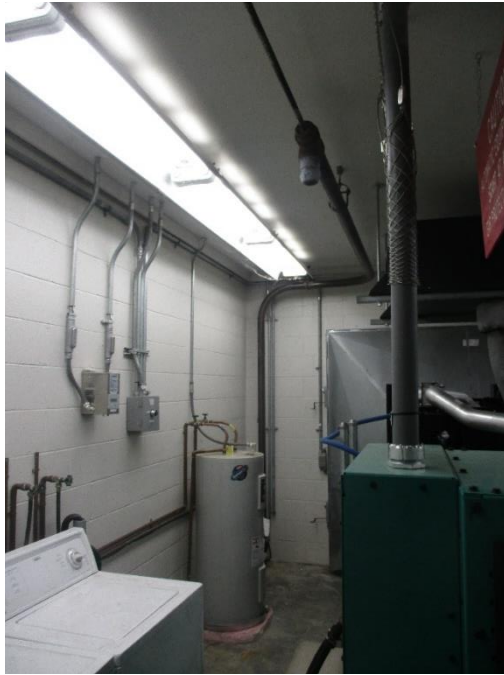
FIGURE B-3 Natural Gas Piping
