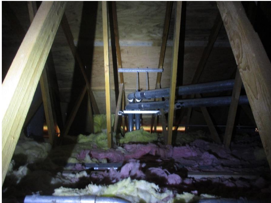
FIGURE B-8 Conduit Runs
