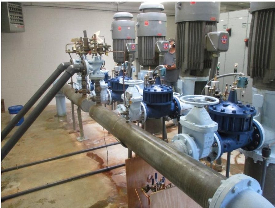
FIGURE B-4 Fluid Piping
