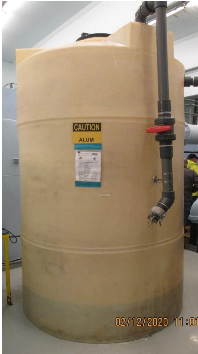
FIGURE A-1 Existing Alum Storage Tank
