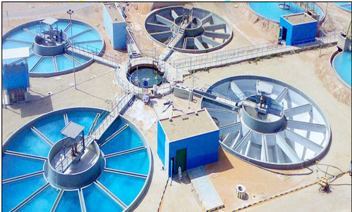
Figure 1. Wastewater Treatment Plant
