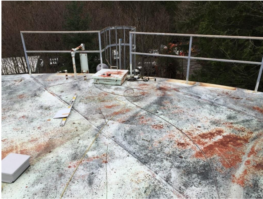
Figure 6 Roof at Entry Hatch
