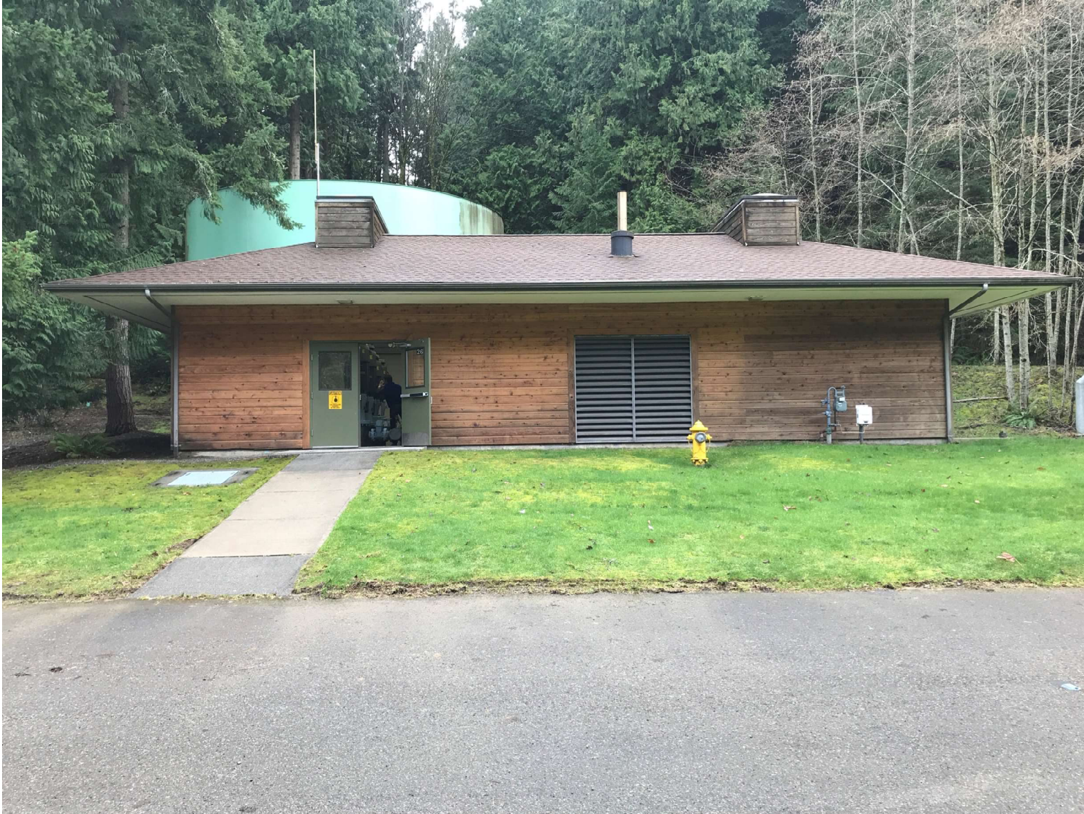
Photographed: Finished Water Pump Building north façade.
