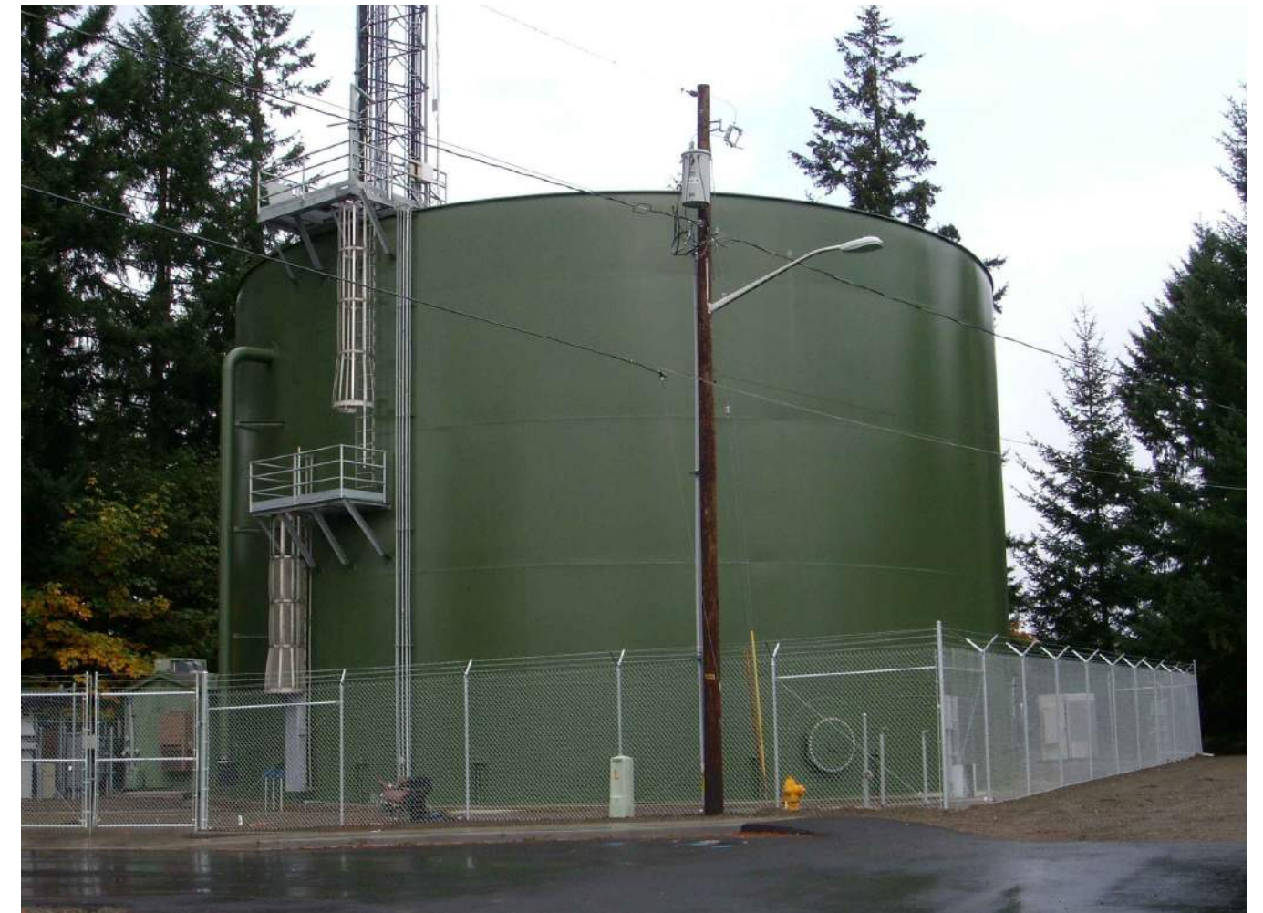
WELDED STEEL RESERVOIR PHOTO SOURCE: GRAY & OSBORNE
