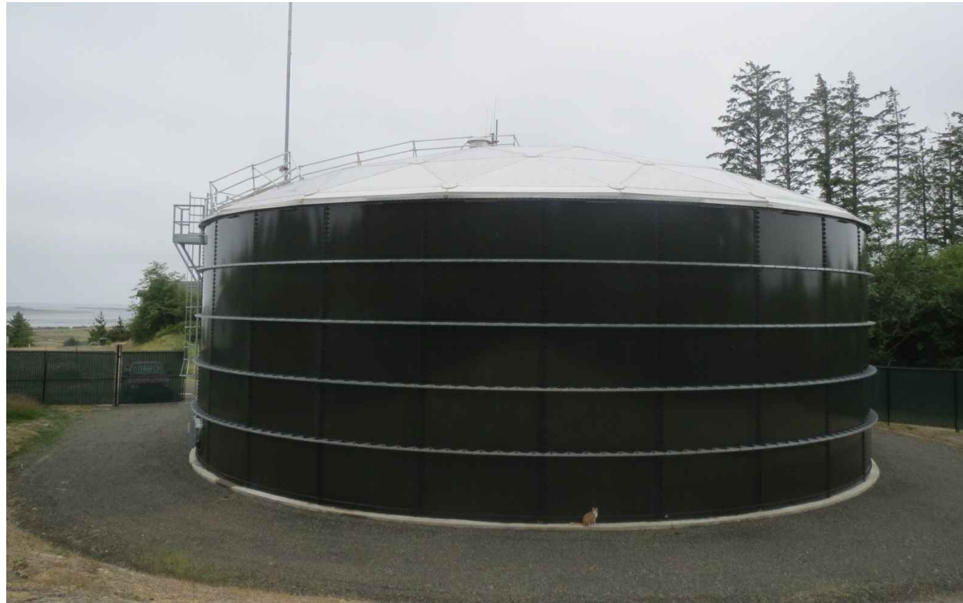
BOLTED STEEL RESERVOIR PHOTO SOURCE: GRAY & OSBORNE
