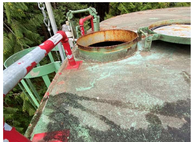
Ladder transition area.
