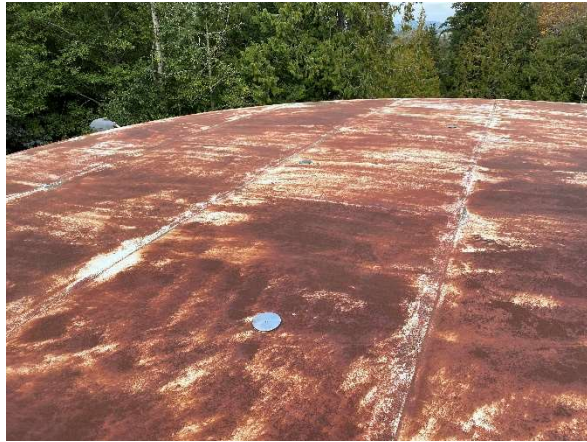
Roof condition in 2022.
