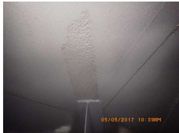
Two examples of the corrosion damage to the roof plates above the rafters of a 38-year-old reservoir.
