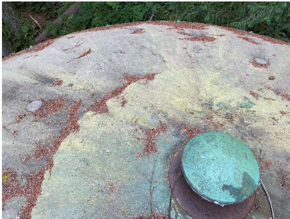
General roof condition.
