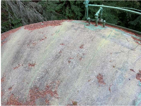
General roof condition.
