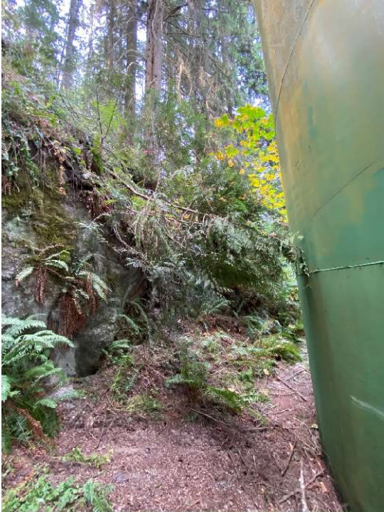
Ringwall below grade.
