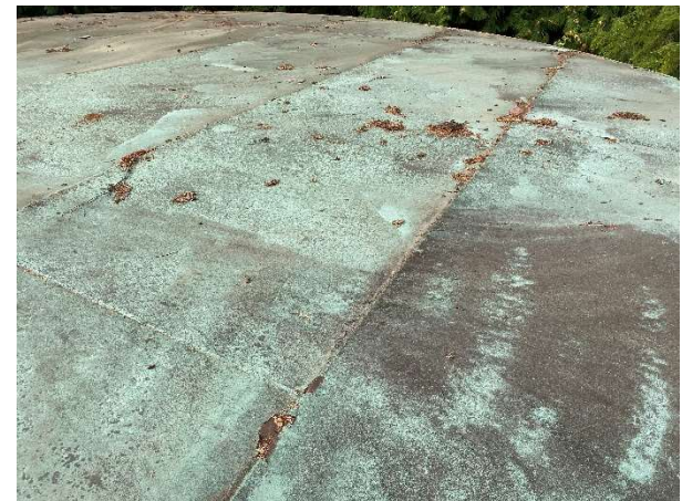
General roof condition.
