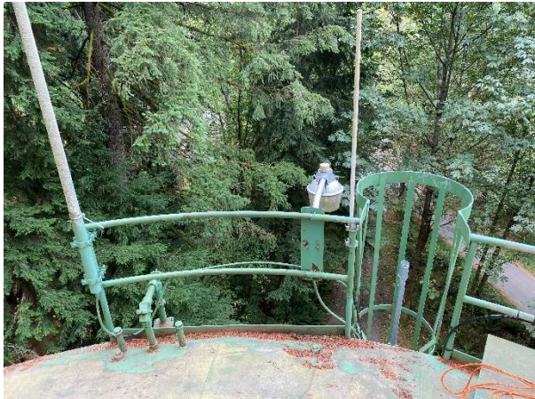
Ladder transition area.
