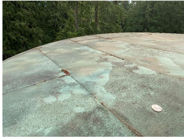
General roof condition.
