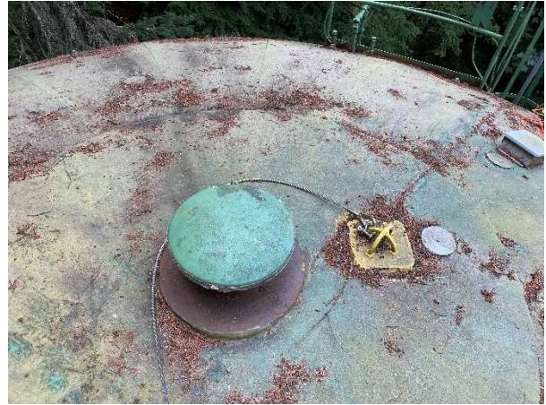
General roof condition.
