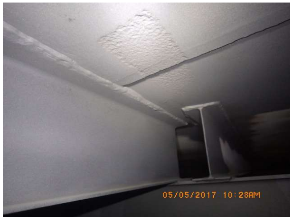
Two examples of the corrosion damage to the roof plates above the rafters of a 38-year-old reservoir.
