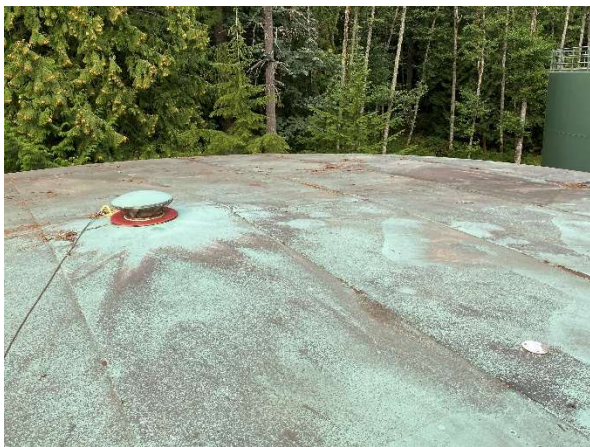
General roof condition.
