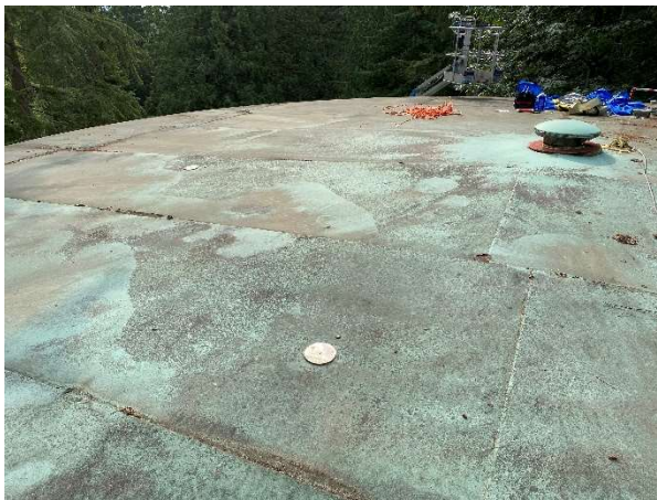
General roof condition.
