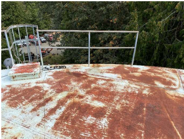
Ladder transition area.
