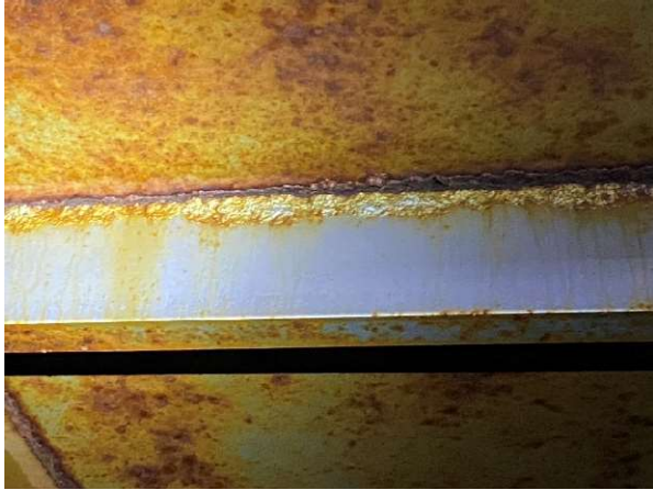
Rafter corrosion.
