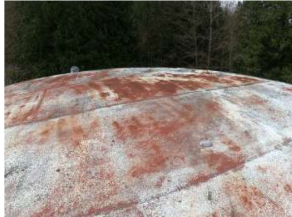
Roof condition in 2018.
