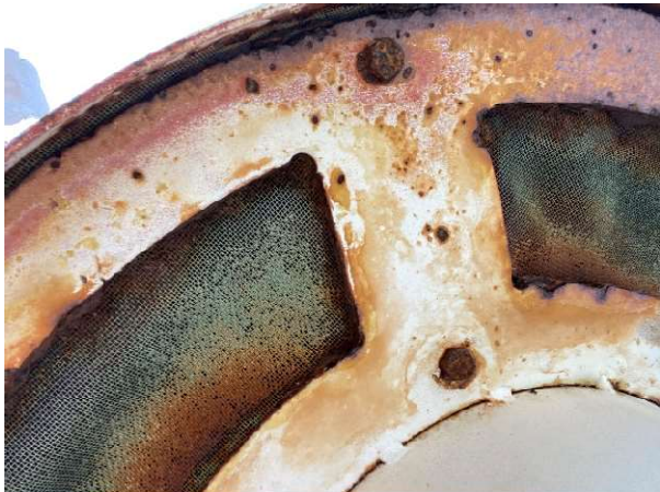
Underside of roof vent.
