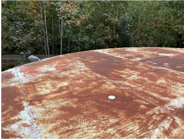
General roof condition.
