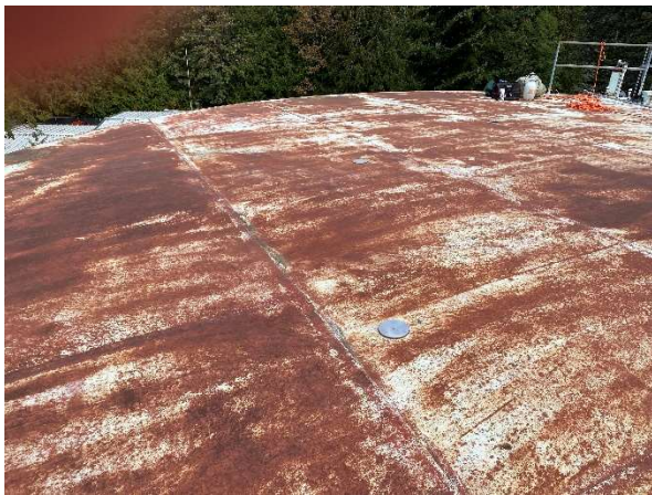
General roof condition.
