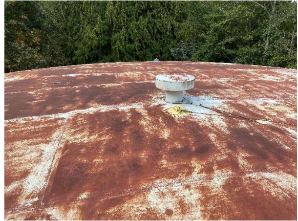
General roof condition.
