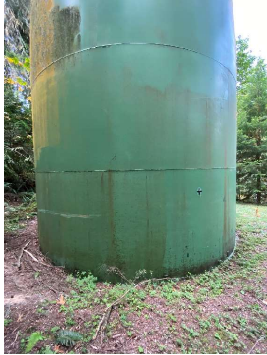
Ringwall below grade.
