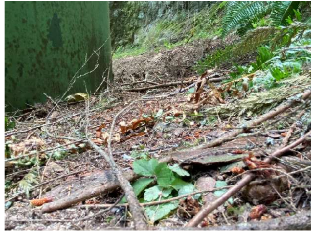
Grade behind reservoir.
