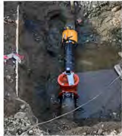
2 6" GATE VALVE - AS-BUILT NOT TO SCALE
